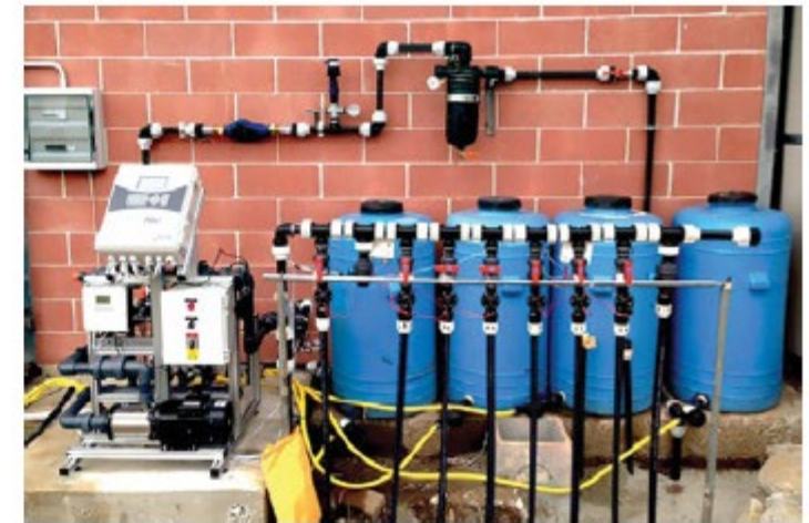
Figure 54. Highly automated fertigation bank (From: Agricoplast website).
